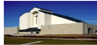
2005 ABC Excellence in Construction Award Associated Builders & Contractors, Inc. Oklahoma Chapter
